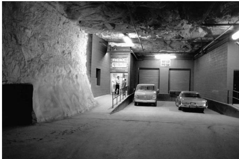
The loading dock and entrance to the high-security Records Center of Kansas City facility, constructed against the side of one of the many massive limestone pillars that were left during mining operations to support the limestone roof of the mine. The Records Center is in the Hunt Midwest Underground complex, which has its own security force and fire department.
