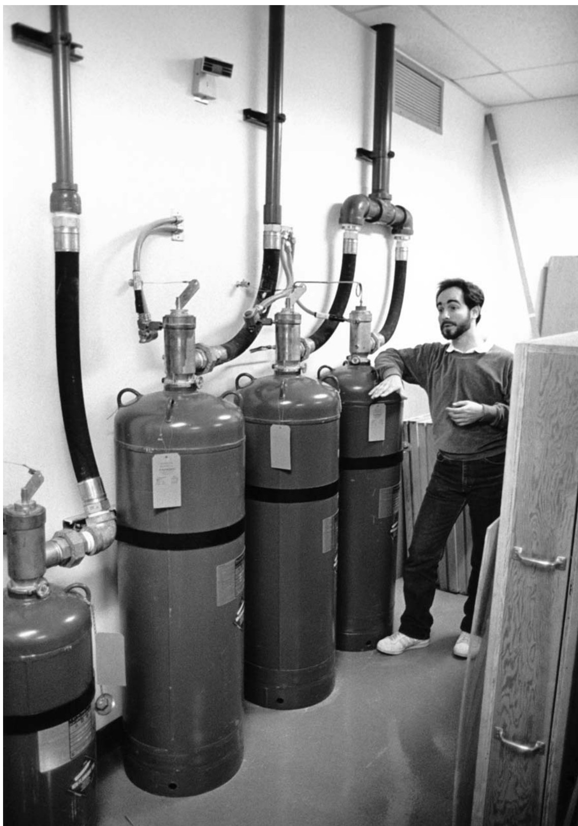
Curator John H. Lawrence is seen here with large cylinders of Haylon gas at the Historic New Orleans Collection in New Orleans, Louisiana. Haylon fire-suppression systems are particularly appropriate for photographic storage areas because, unlike water or other liquid and dry chemical fire extinguishers, Haylon gas does not freeze, leaves no residue, and does not harm photographs, paper, or other fragile materials.
