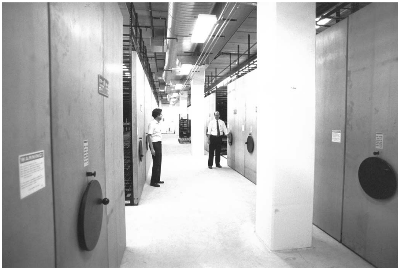
One of the three film storage vaults in the new Warner Bros. high-security motion picture cold storage building on the Warner Bros. studio lot in Burbank, California. The color film vault, which is maintained at 35°F (1.7°C) and 25% RH, and the other vaults were operating and in the final phase of testing when this photograph was taken on October 8, 1992. Warner Bros. began moving its film collection into the vaults a few weeks later. Shown here in the larger black-and-white film vault, which, like the two other vaults in the building, is equipped with movable shelving that permits high-density film loading, are John Belknap, manager of Film Vaults/Assets, and Bill Hartman, manager of Asset Inventory Management and Research in Corporate Film Video Services at Warner Bros. The $9-million cold storage facility was designed under the direction of Peter R. Gardiner, vice president of Operations in Corporate Film Video Services at Warner Bros. (a division of Time Warner Inc.). See Chapter 9 for additional discussion of the film preservation program at Warner Bros.
