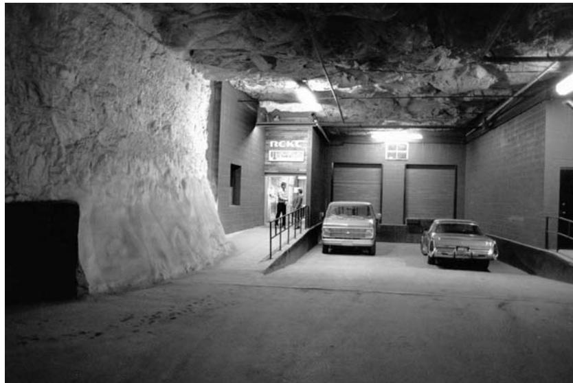
The loading dock and entrance to the high-security Records Center of Kansas City facility, constructed against the side of one of the many massive limestone pillars that were left during mining operations to support the limestone roof of the mine. The Records Center is in the Hunt Midwest Underground complex, which has its own security force and fire department.
