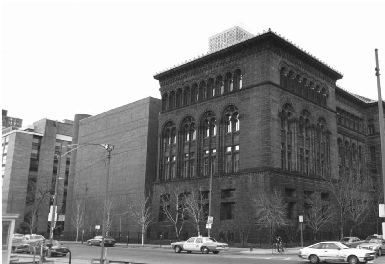
The Newberry Library, founded in 1887 in Chicago, is one of the country's leading research libraries. The temperature- and humidity-controlled bookstack building, completed in 1982, is the windowless structure located behind the main library building. Fireproof passageways provide access to each floor from the main library.
