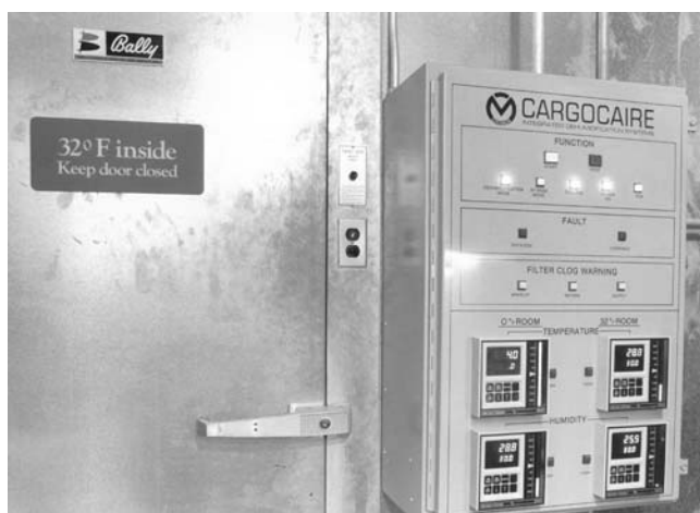
The 0°F vault for nitrate film storage is located inside the larger 32°F vault. The control panel on the right monitors temperature and humidity levels in both vaults.
