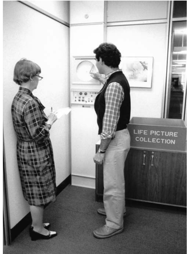
Temperature and humidity conditions inside the vault are recorded on a circular chart recorder, here being checked by Mary Jane McGonegal and George Zeno.
