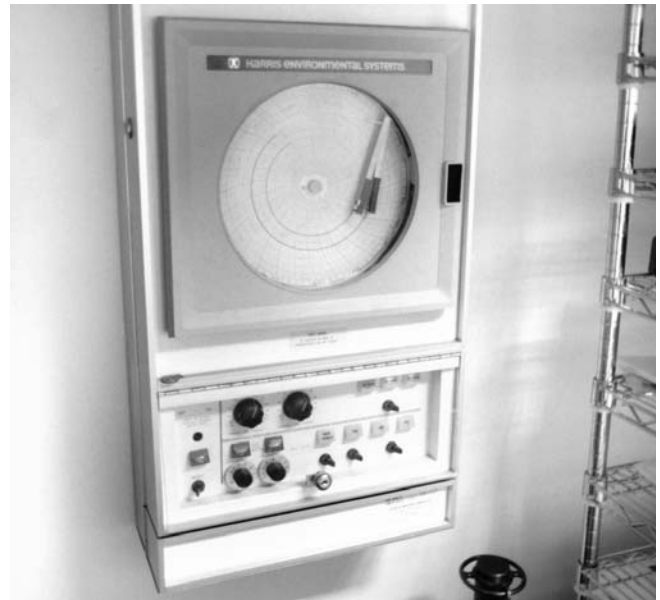
One of the two vault control panels, located near the vault entrance. The temperature and humidity levels are continuously recorded on circular paper charts. Alarms sound and a fail-safe control system automatically shuts down the vault dehumidifiers and refrigeration compressors if either the temperature or relative humidity deviates beyond pre-set limits. The facility was designed and built by Harris Environmental Systems, Inc.
