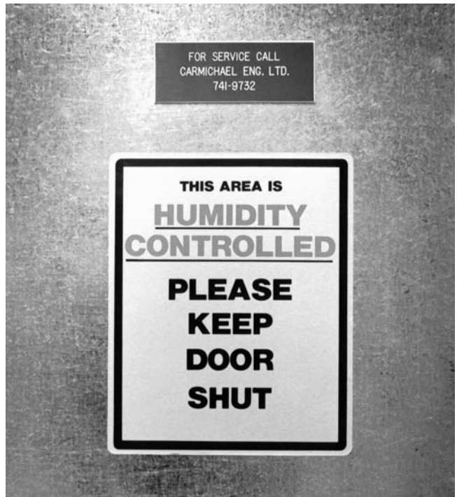
Sign on the vault door. A study conducted by the Film Section of the Moving Image, Data and Audio Conservation Division in Ottawa showed that it was far less expensive and much less labor-intensive to control the humidity in the vault than it would be to pre-condition and package films in vapor-proof bags for storage in a vault with uncontrolled humidity.
