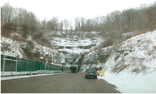
The guarded entrance to the Iron Mountain/National Underground Storage Vital Records facility, located in a secluded area about an hour's drive northeast of Pittsburgh, Pennsylvania.
